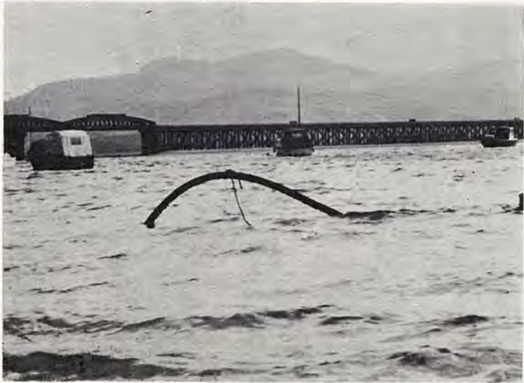
At full tide, the cable safely lifted and harnessed.
